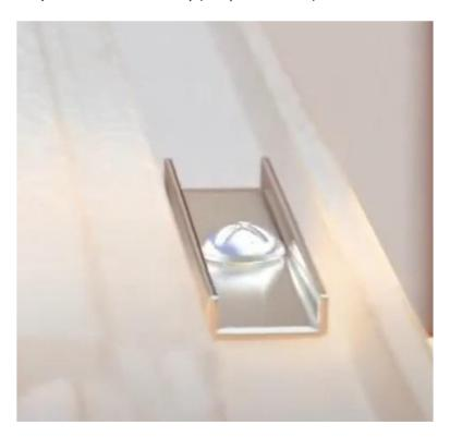
• DO NOT use any silicone/fix-all <u>until</u> the process is complete, afterwards run a layer of silicone around whole way around where your sheet meets your U-profiles and compress so that it is all the one sealed unit.
